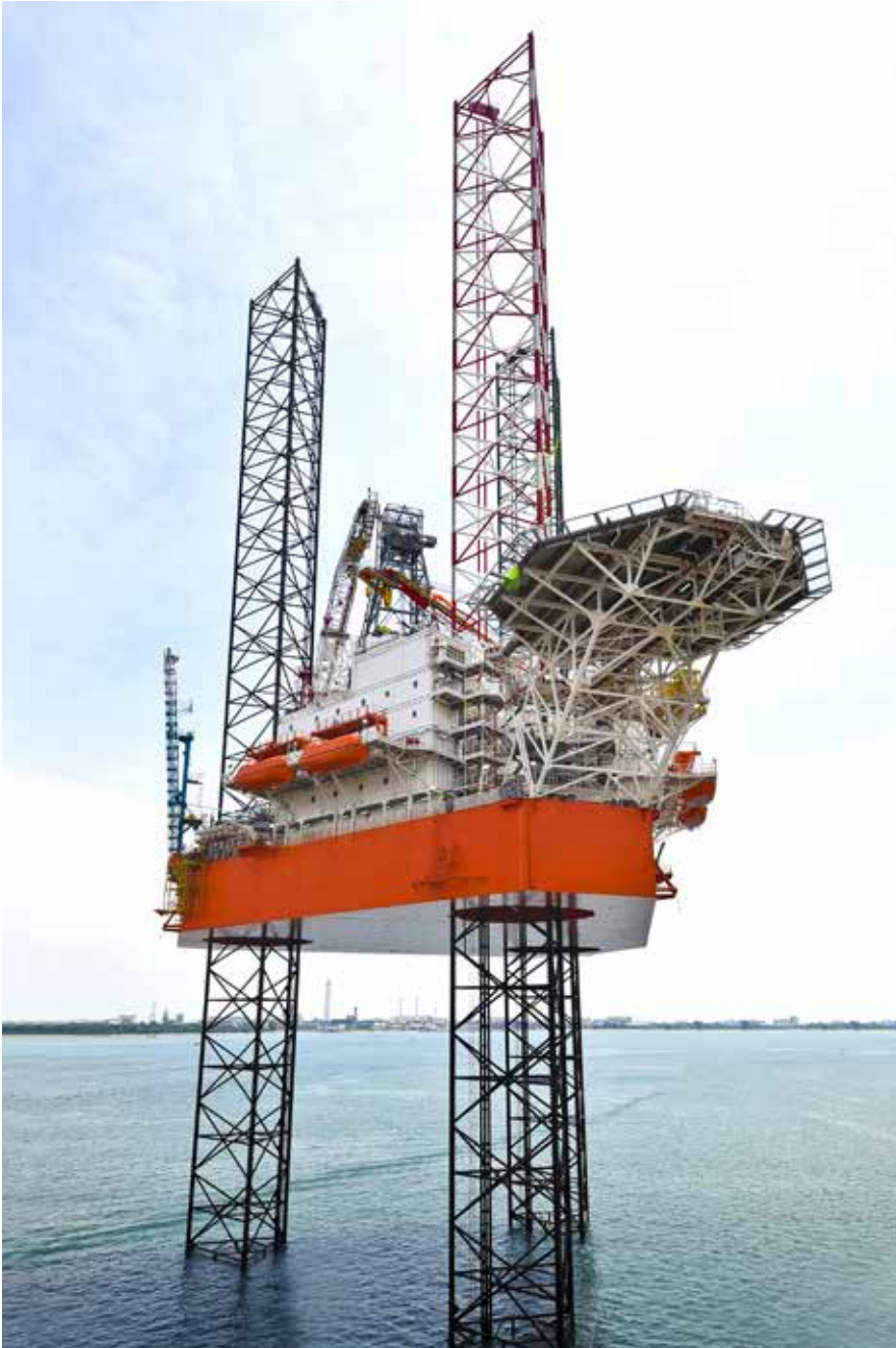
Keppel O&M delivered its first rig of 2020, Heimdal, on 15 January 2020
