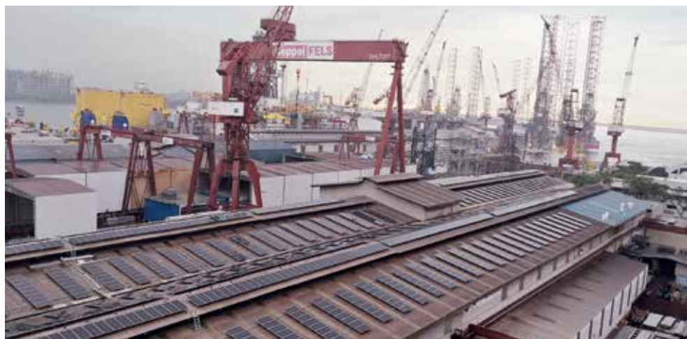
Solar panels laid out at Keppel O&M's yard
